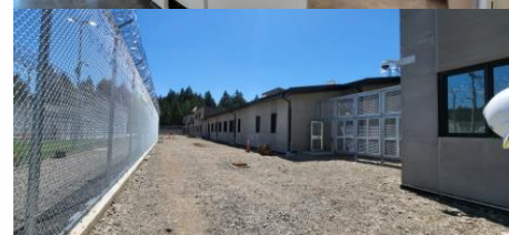
The new (95% completed) NW Joint Regional Correctional Facility
